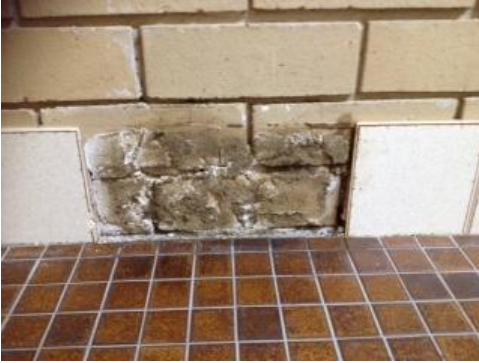
Missing tile in Men's Showers
