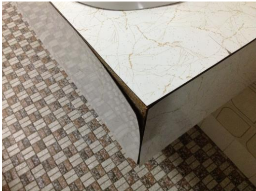
Laminate old and broken
