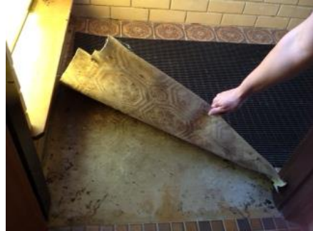
Concrete hallway floor
