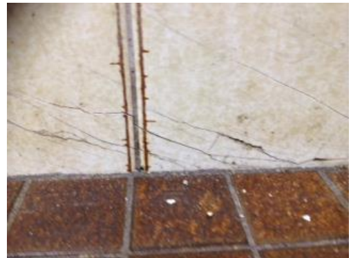
Cracked tiles in Men's Showers
