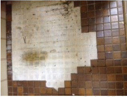
Broken/Missing tiles in Ladies' home showers
