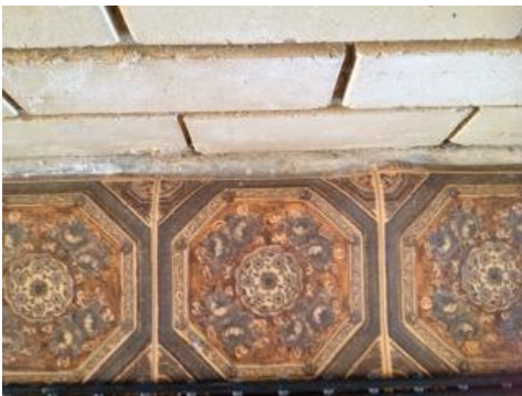
Concrete hallway floor covered in unstuck laminate
