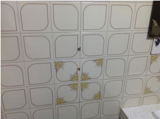
Holes in wall
