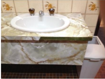
Broken laminex on ladies' toilet vanity
