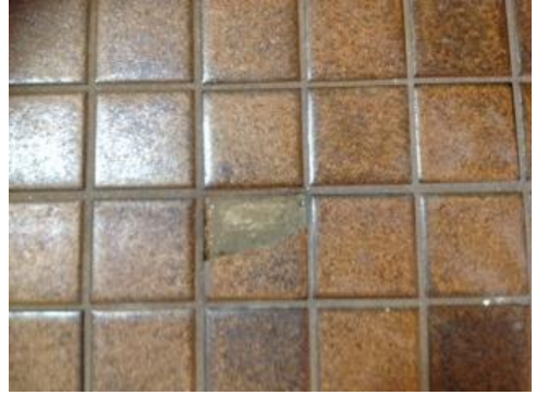
Cracked tile in Men's Shower
