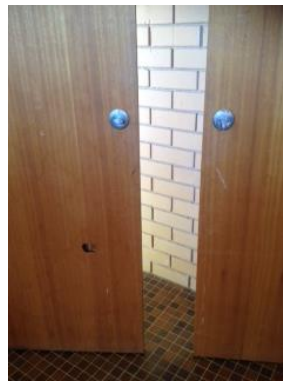
Damaged internal doors – missing handles and hole
