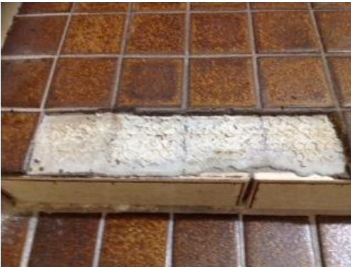
Missing tiles in Men's Showers
